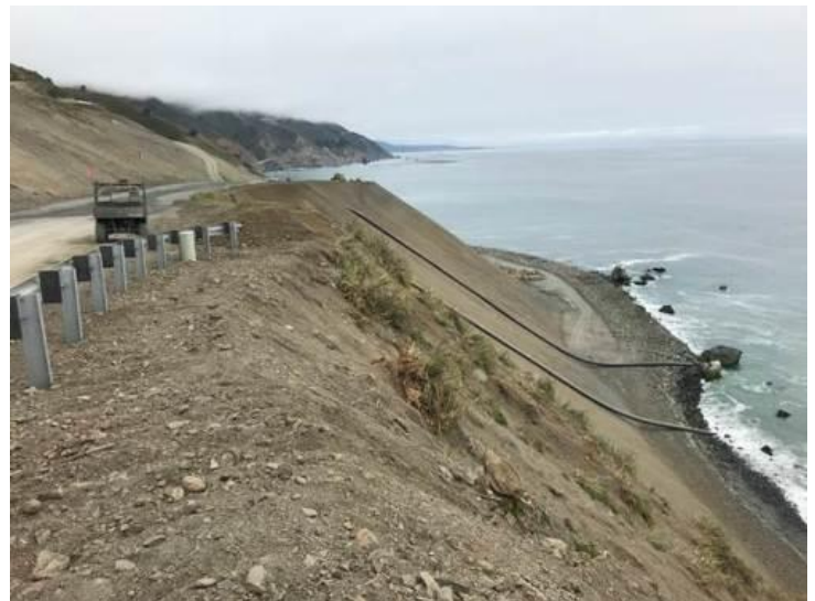
Highway 1 at Mud Creek near Gorda, looking south. Photo courtesy of Caltrans.
