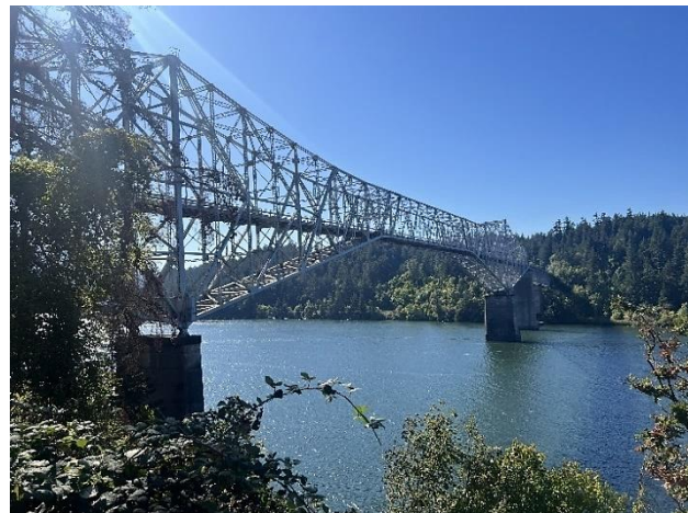
The Bridge of the Gods crossing the Columbia River
